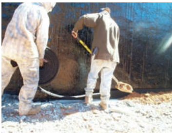
Unrolling Bottom Drain
