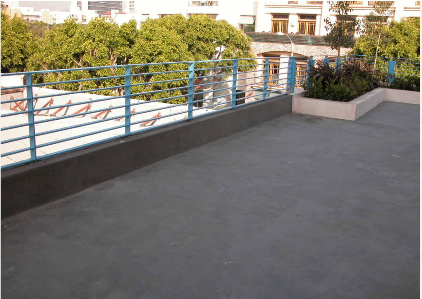
INSTALLATION AVM SYSTEM 100 FOREVERCOAT
