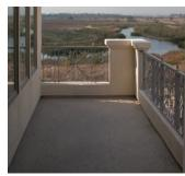
**Step 5:** Top Coat: Apply the AVM 680SC Aliphatic Top Coat (U-680SC-ALTC) by roller, spray or squeegee followed by back rolling, in one uniform coat at minimum rate of 100 sq.ft./Gal in order to obtain a minimum coating thickness of 16 wet mils and to completely coat the aggregate.
