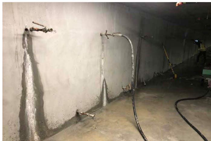
FIG. 2 - INJECTION PORT LAYOUT
