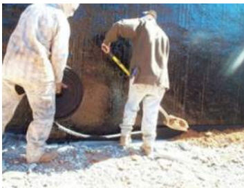
Unrolling Bottom Drain
