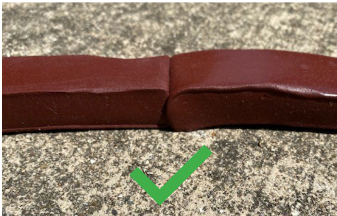
FIG 2. - AUSSIE SWELL RED TIGHTLY BUTTED TOGETHER
