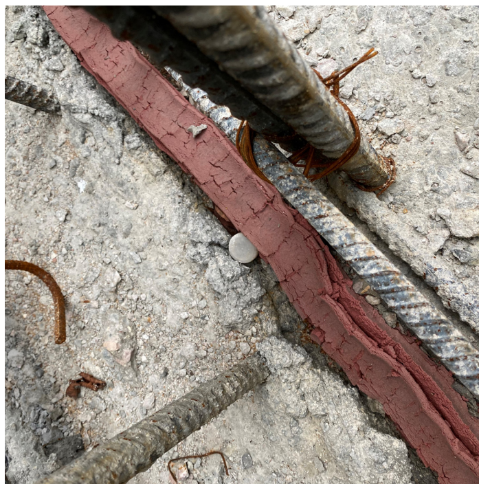
FIG. 7 – PRE-HYDRATED AUSSIE SWELL RED NEEDING REMOVAL
