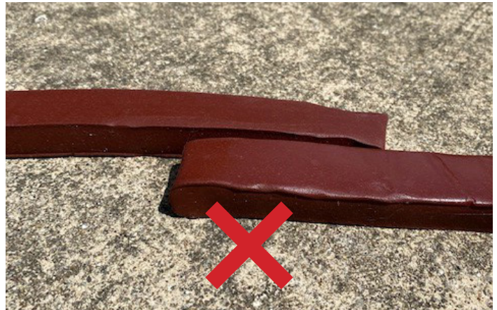
FIG 3 - ENDS OVERLAPPING INSTEAD OF BUTTED. NON-COMPLIANT.
