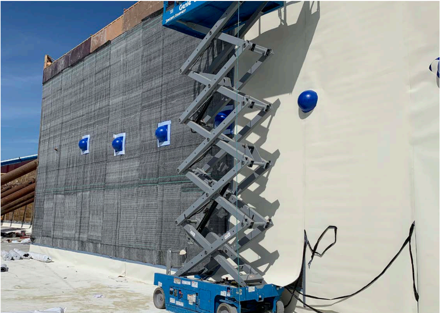
FIG 1 – AUSSIE SKIN 550 INSTALLED ON BLINDSIDE WALL
