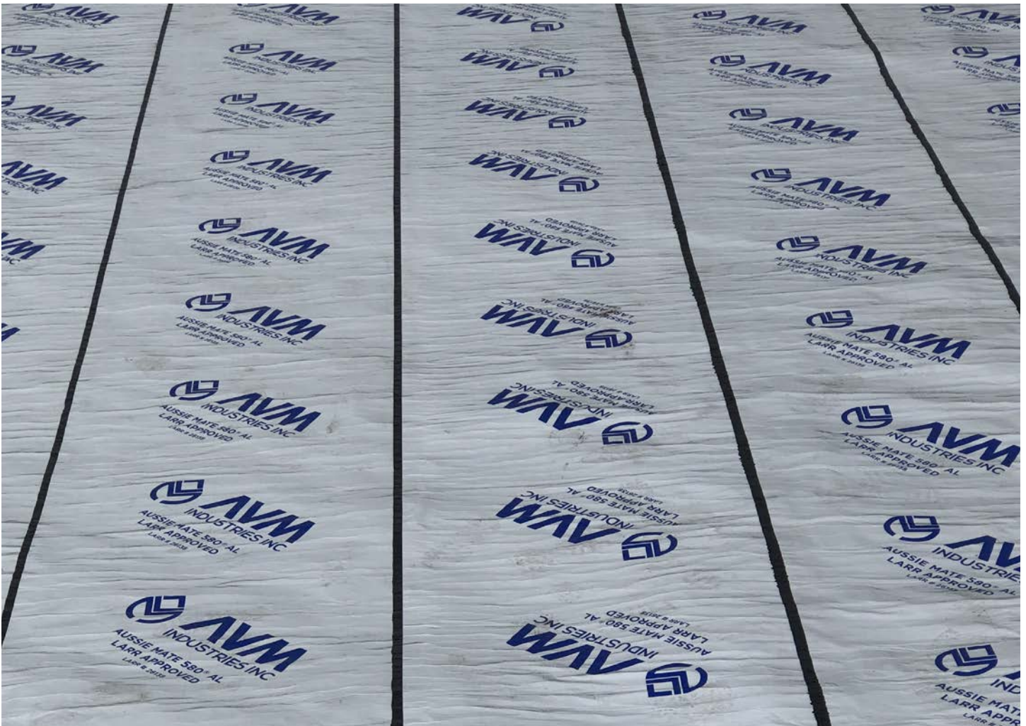
FIG 1 - AUSSIE MATE 580-AL INSTALLED HORIZONTALLY
