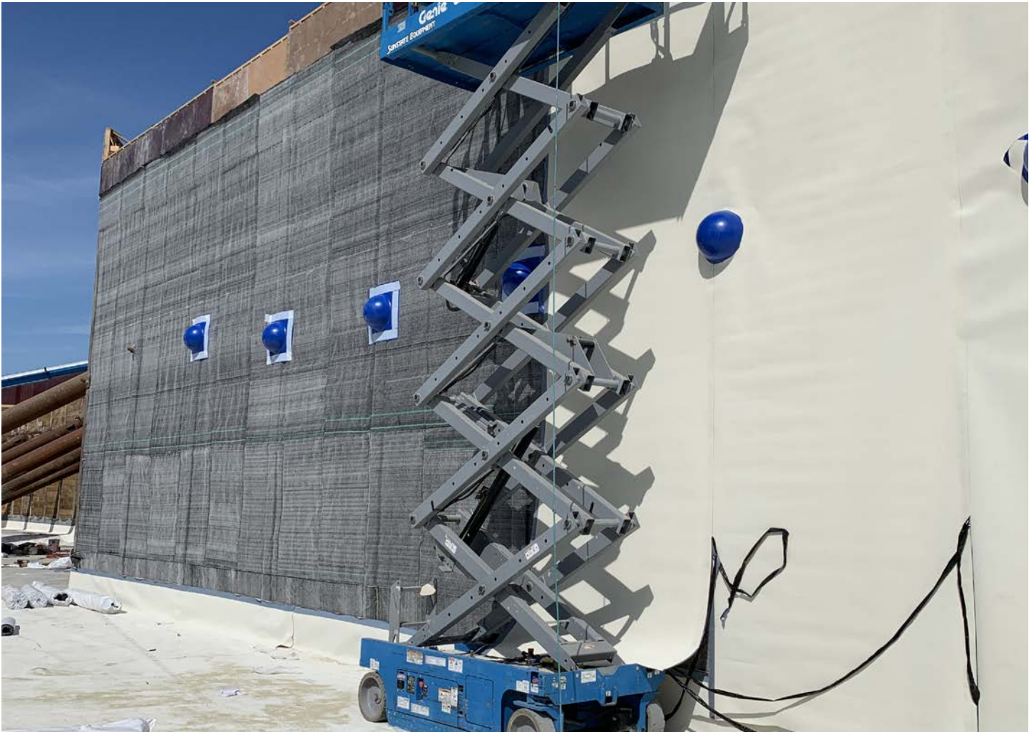
FIG 1 – AUSSIE SKIN 550 INSTALLED ON BLINDSIDE WALL
