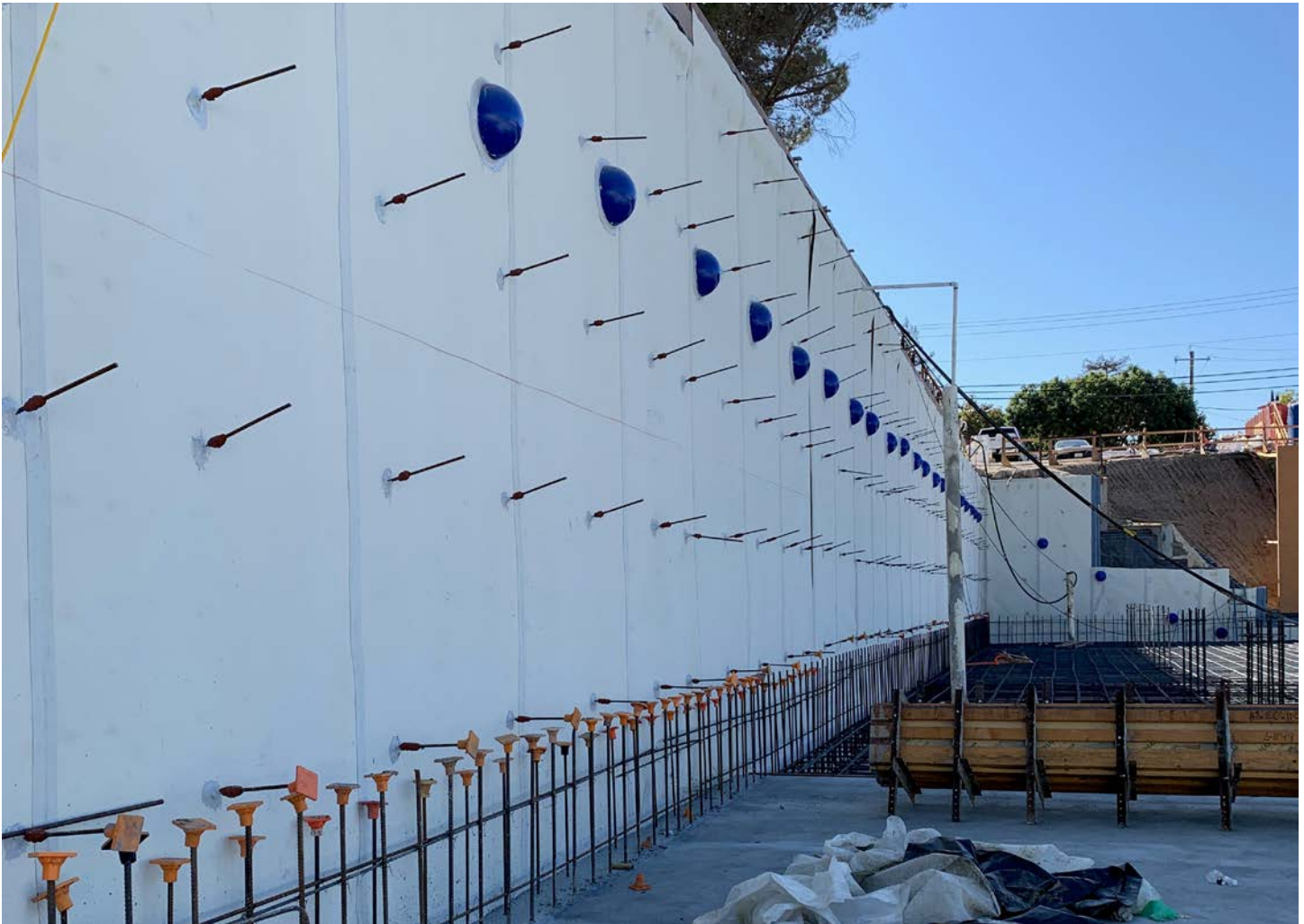
FIG 1 – AUSSIE SKIN 560G INSTALLED ON BLINDSIDE WALL
