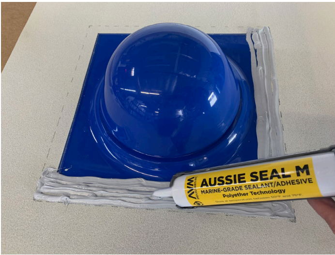
Step 9: Apply Aussie Seal M sealant 1" onto the Aussie Skin and 1" onto to the Cone's base.
