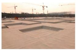
7. In areas where formwork is to be removed (slab edges, footings, top of wall) for tie-in to post-applied waterproofing, the formwork shall remain in place for a minimum 72 hours after placement of concrete. Please contact AVM if form removal is scheduled sooner as this could affect the Aussie Skin's bond to the concrete.
