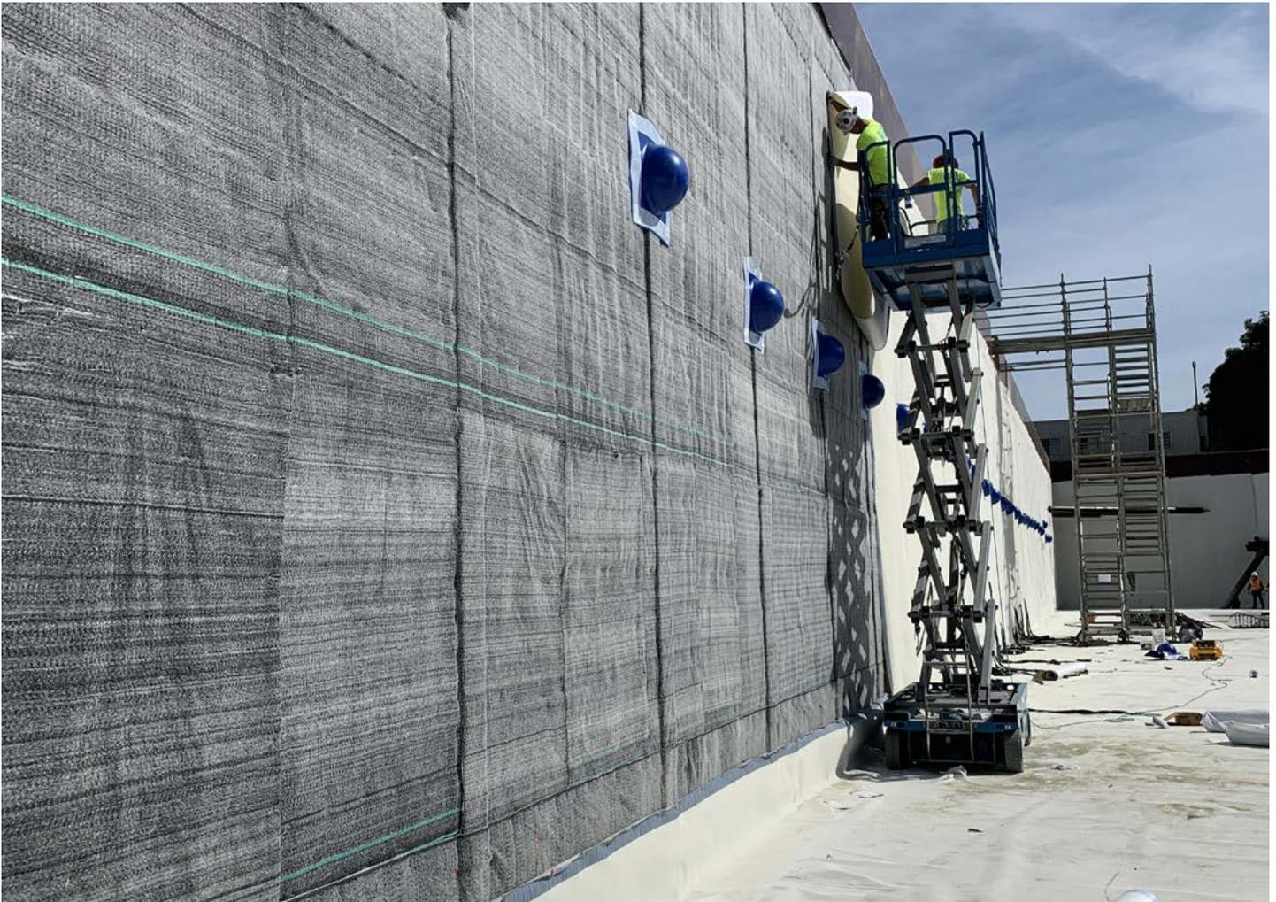
FIG 1 – AUSSIE SKIN 560G INSTALLED ON BLINDSIDE WALL
