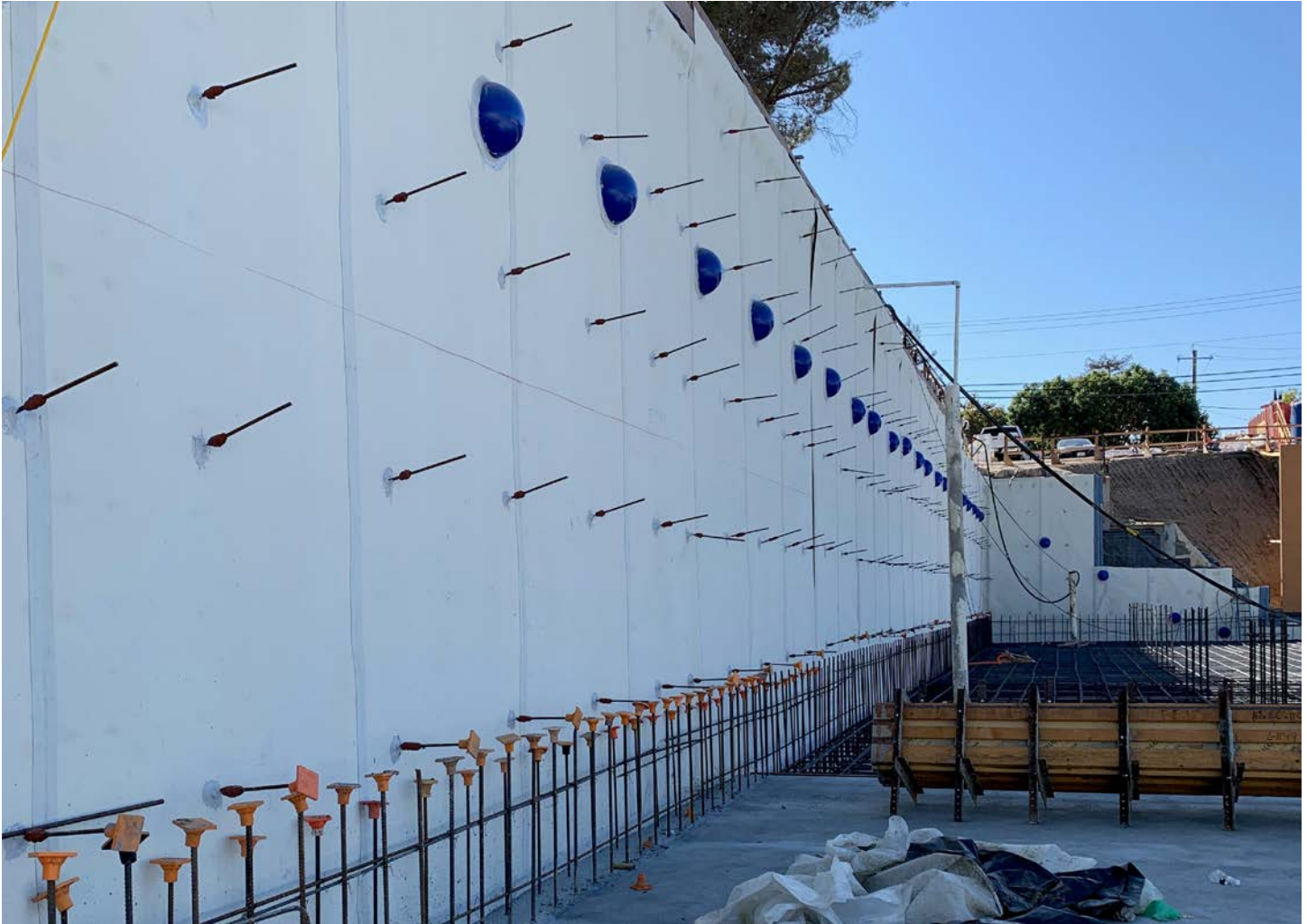
FIG 1 – AUSSIE SKIN 560G INSTALLED ON BLINDSIDE WALL
