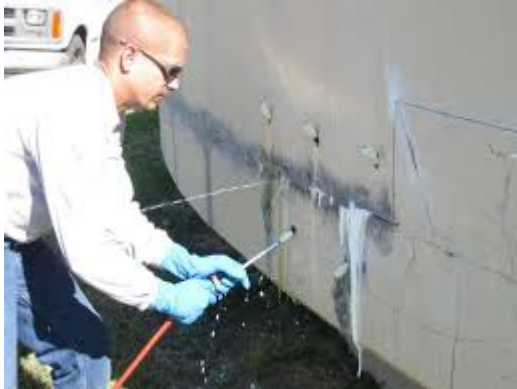
Fig. 5 - Injection of Urethane Resin
