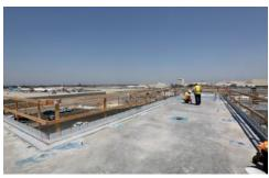
PSI: On traffic bearing surfaces, concrete substrates shall achieve a min compression strength of 2000 psi prior to installation.
