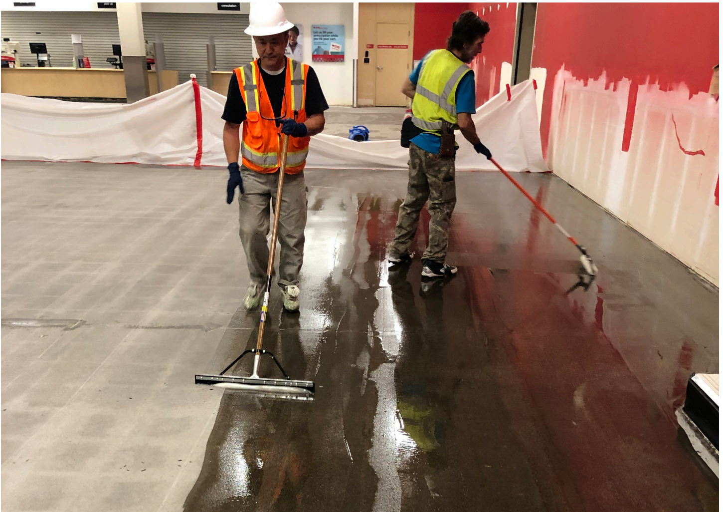
INSTALLATION OF AVM GAS-LOCK® 420
