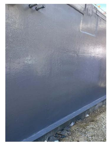
Figure 1b: Second and final coat of Aussie Membrane 520 PRO is completed and expected to be fully cured in 24-48 hours.
