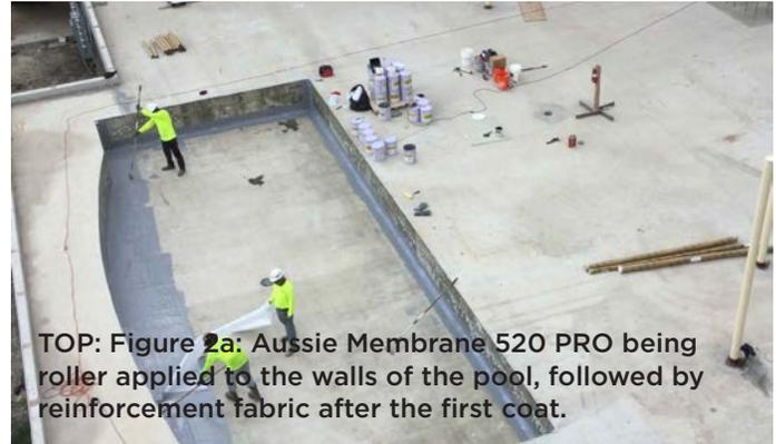
TOP: Figure 2a: Aussie Membrane 520 PRO being roller applied to the walls of the pool, followed by reinforcement fabric after the first coat.
