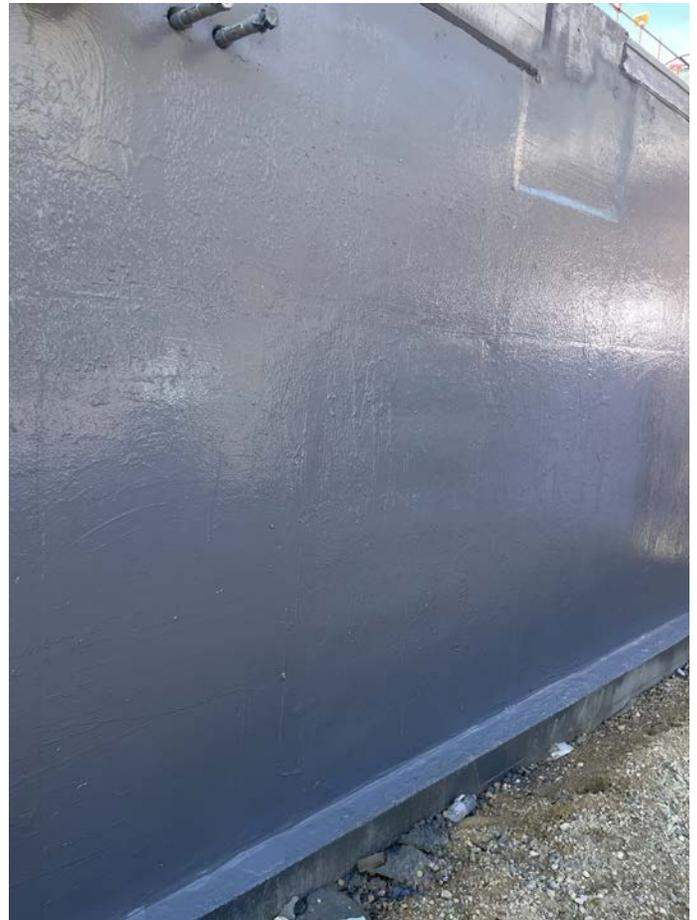
Figure 1b: Second and final coat of Aussie Membrane 520 PRO is completed and expected to be fully cured in 24-48 hours.
