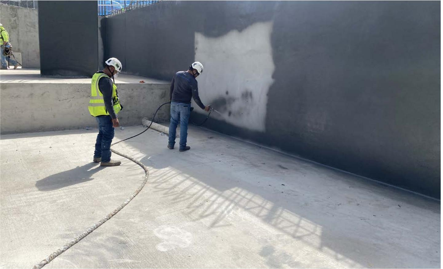
Figure 1a: Applicator spraying the first coat of Aussie Membrane 520 PRO in the post applied wall application, using Graco pump approved for polyurethane coatings.
