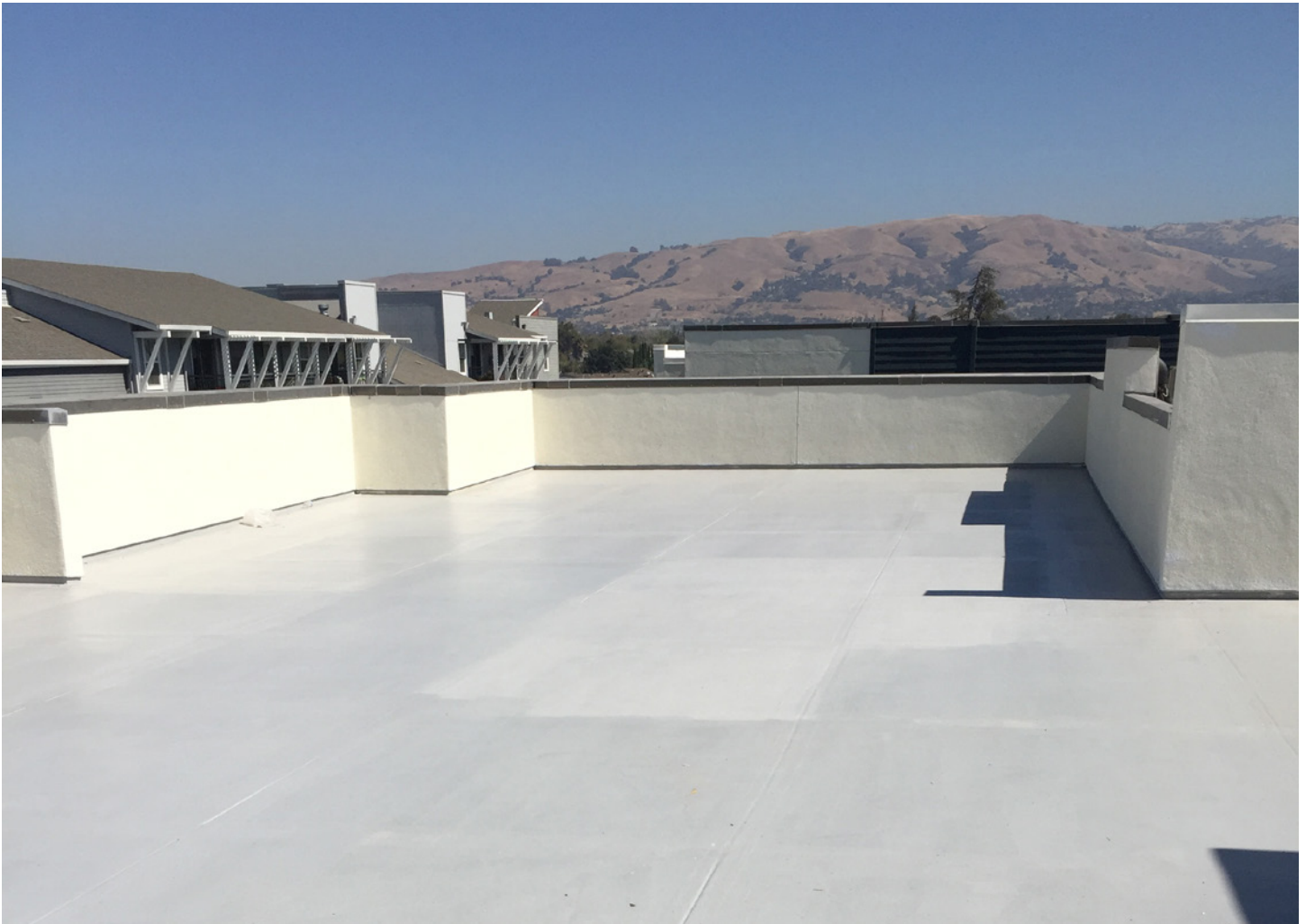
INSTALLATION AVM SYSTEM 100 ELASTO FIBERDECK
